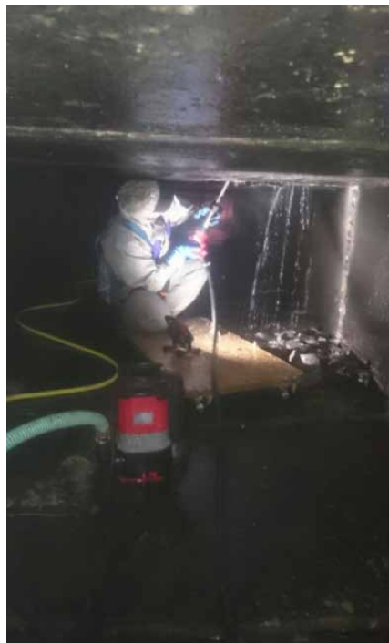
The Bawax applicator cleans an overhead joint between precast segments of the box culvert to provide a clean space for the application of Xypex Patch'n Plug.
