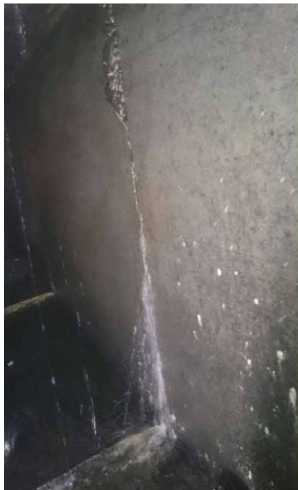
Every joint between segments of the precast box culvert was leaking prior to the repair project. It is estimated that more than 1.7 million liters per day was leaking into the culvert from the Oese River, which flowed just above the structure.
