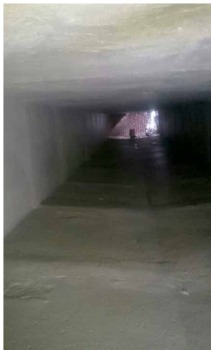
Culvert coated with Xypex Concentrate crystalline waterproofing.
