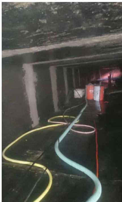
Xypex Patch'n Plug was applied to 102 meters of leaking cracks and joints between segments of the precast box culvert. Here, as the Bawax applicator completes the first phase of the project, most leakage has been halted.
